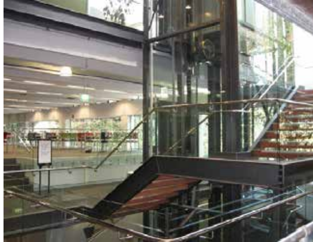
| University Fire & Smoke Compartmentation
