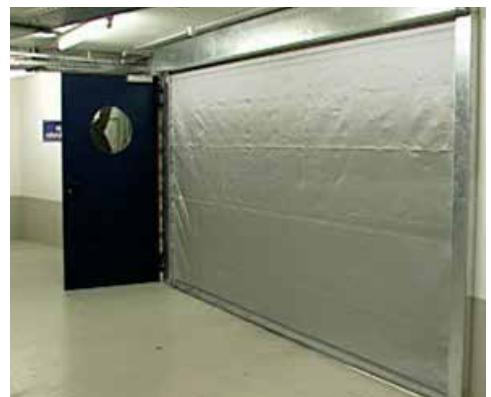
Fire and smoke compartmentation in a basement carpark with additional egress door. An egress door prevents occupants from driving out of the car park and blocking fire fighting activities
