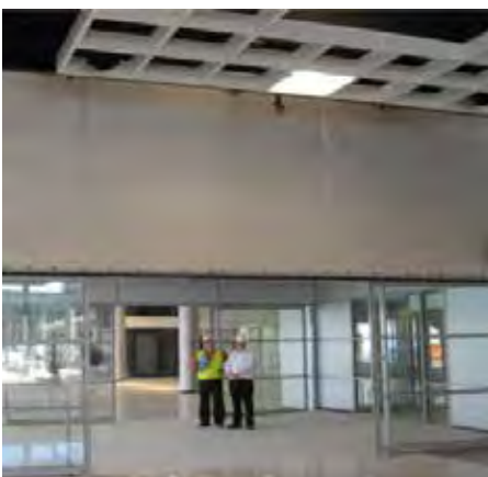
Fibershield V protecting an existing installation of non-fire rated glazing
