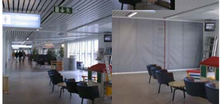
To provide open space, assist with way-finding and to comply with smoke compartment wall requirements in this building, Fiberseal was installed to operate as an automatic smoke wall.
