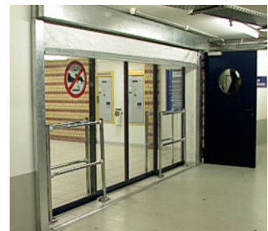
Fiberseal FS fire and smoke containment screen used to separate a carpark from a shopping centre to upgrade existing glazing system. The system has commenced deployment. See full deployment below.
